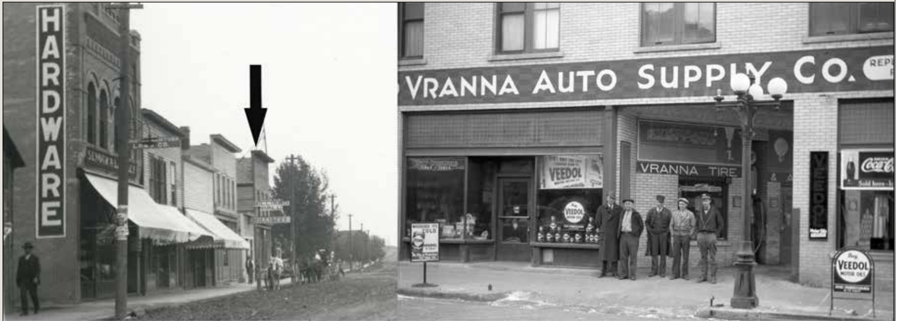
Left: The original woodframe Messersmith building on the corner of Sims and 1st Street. Right: The new brick Vranna Block building with the diagonal cut in on the corner. Images from SWNDDA.
